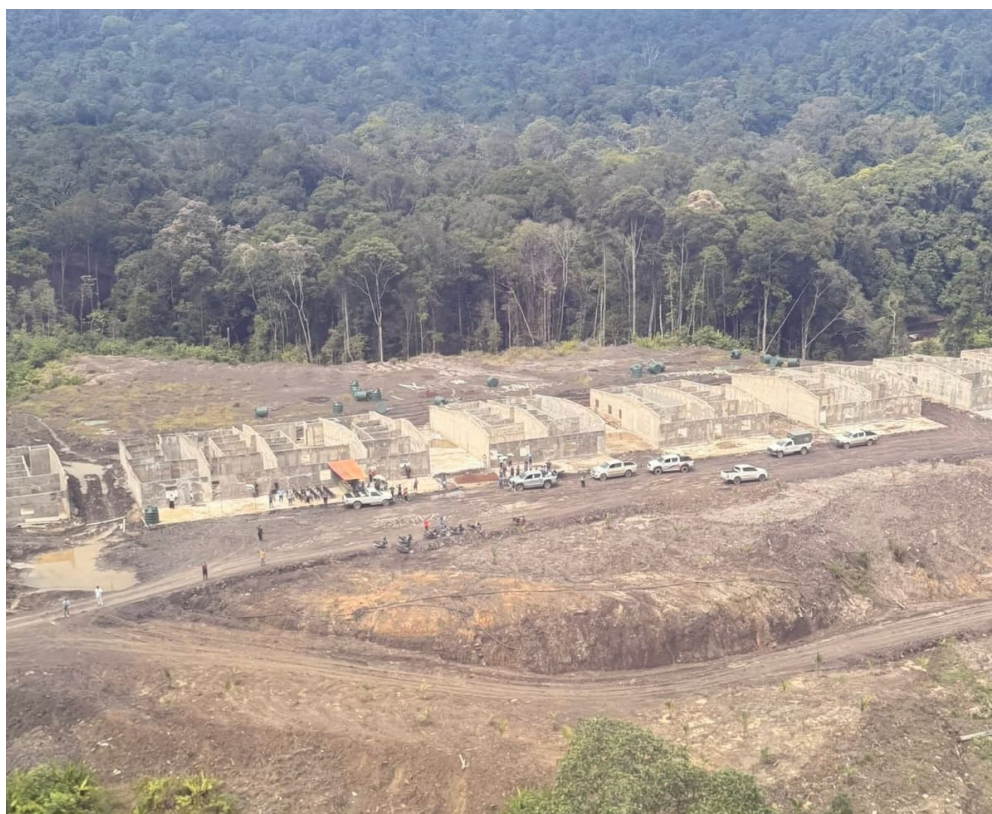
Picture 25: Unfinished brick houses constructed by FDS in Ba Data Bila (Forest Department Sarawak) 121
